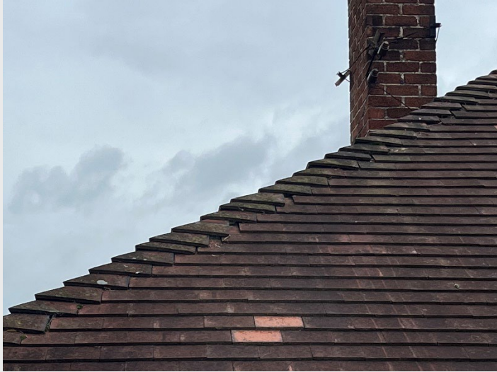
Photograph 21: Slipped tiles along ridge of B4
