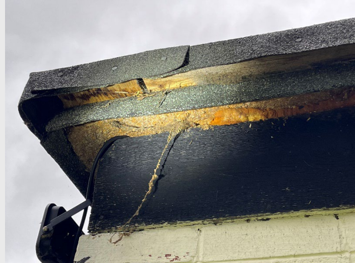
Photograph 14: Gap in roofing within southwestern corner of B1
