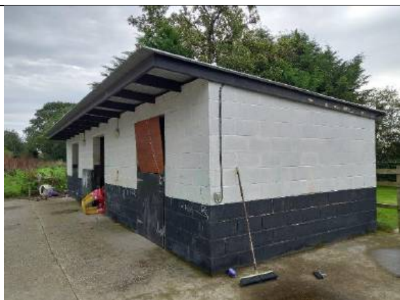
Photograph 14: Stable block (B4b)
