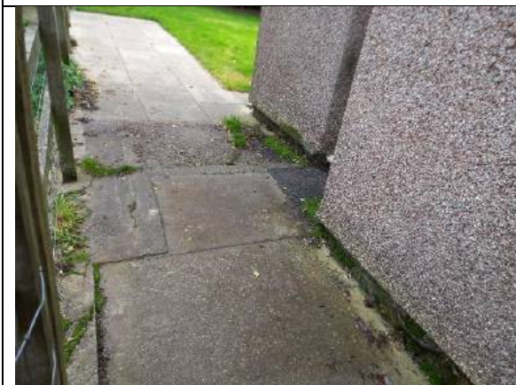
Photograph 3: Paving stone slabs
