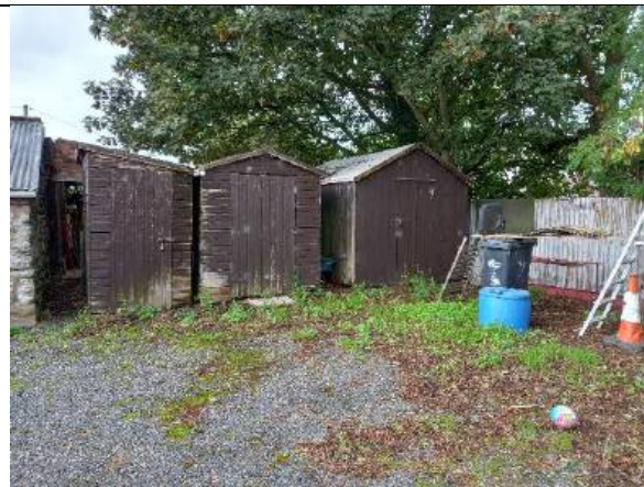
Photograph 34: Timber sheds (TN4)
