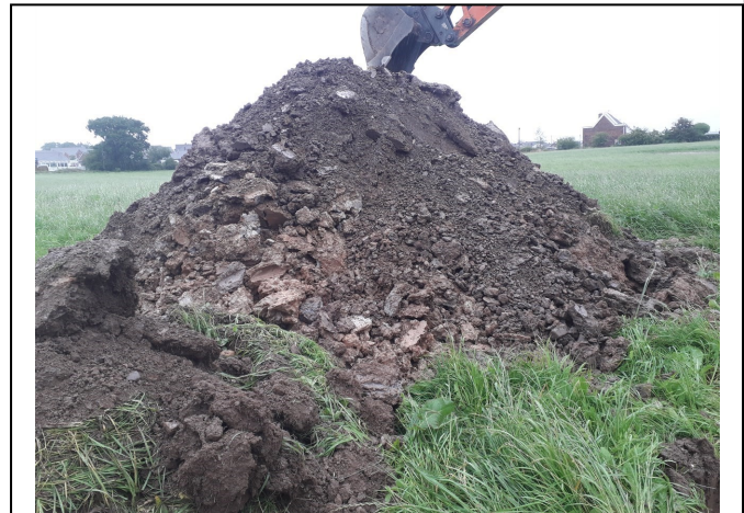
Trial Pit 127 Spoil
