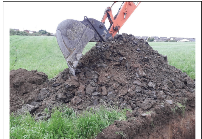
Trial Pit 128 Spoil
