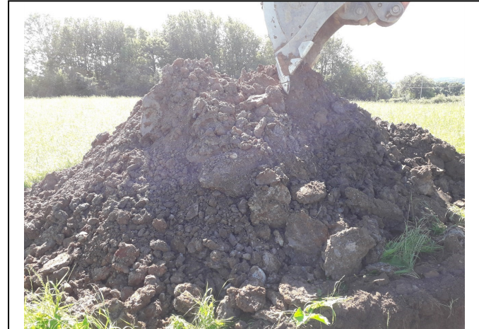
Trial Pit 110 Spoil
