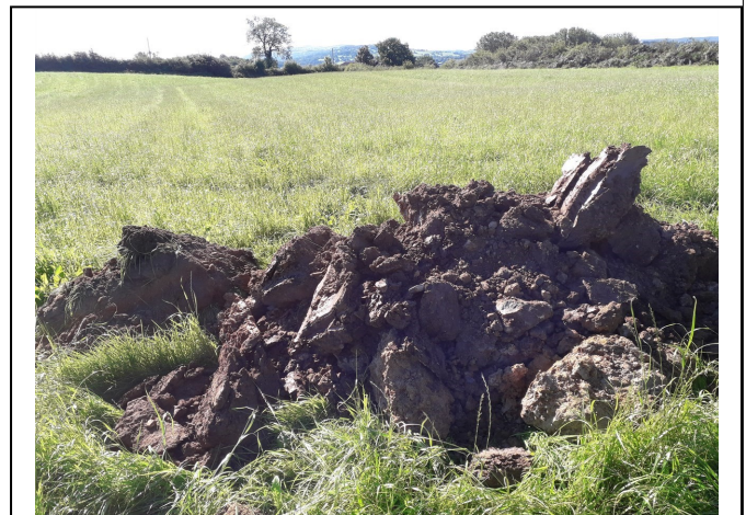
Trial Pit 108/ Soakaway 104
