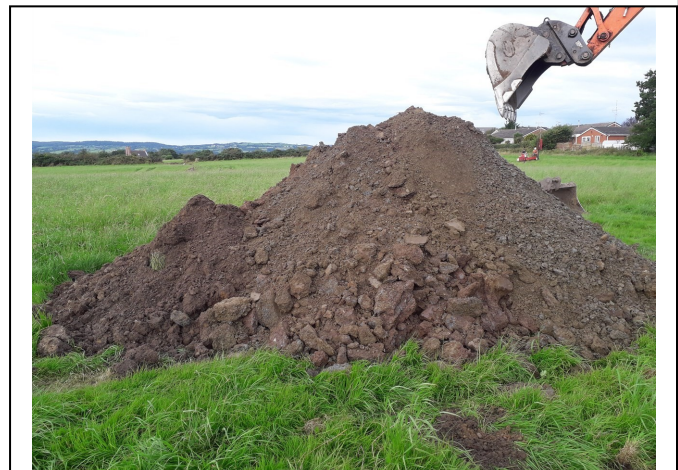
Trial Pit 121 Spoil
