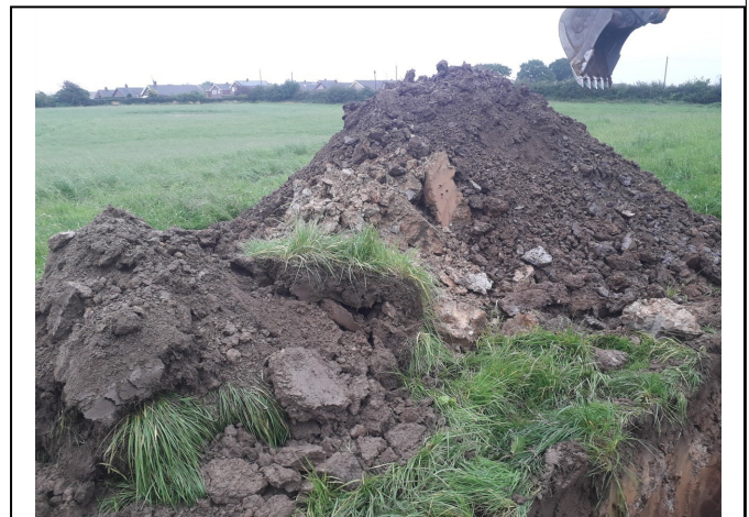
Trial Pit 129 Spoil
