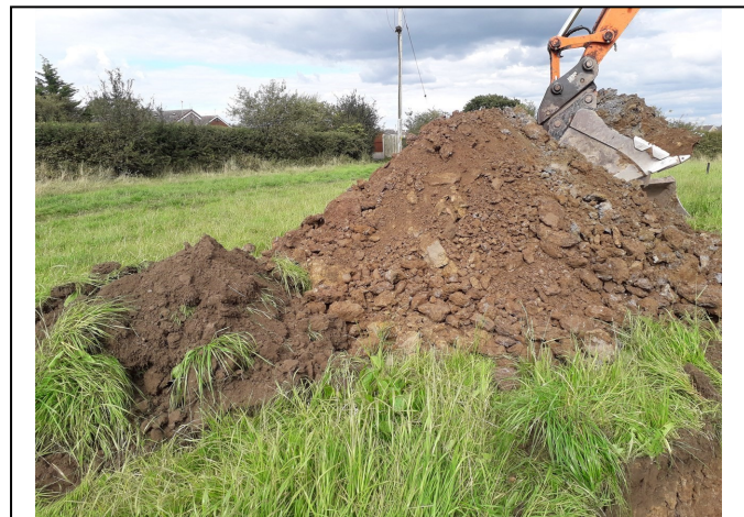
Trial Pit 117 Spoil
