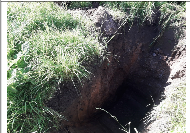
Trial Pit 107/ Soakaway 103
