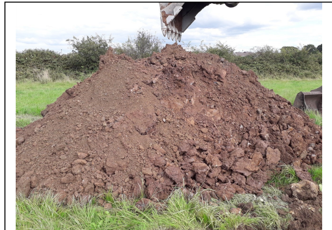
Trial Pit 114 Spoil
