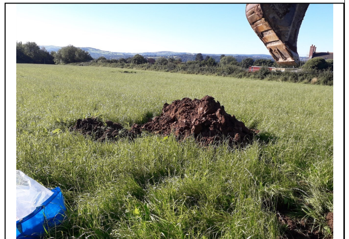
Trial Pit 104 Spoil
