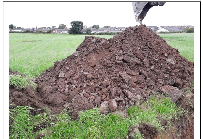
Trial Pit 125 Spoil
