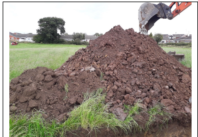
Trial Pit 122 Spoil
