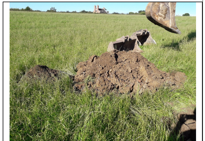
Trial Pit 106 Spoil
