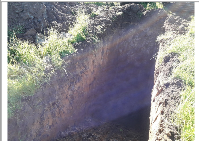
Trial Pit 105/ Soakaway 101
