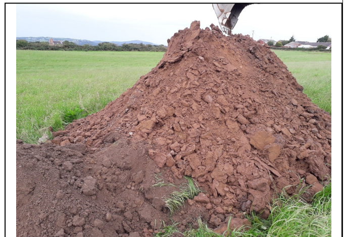
Trial Pit 124 Spoil
