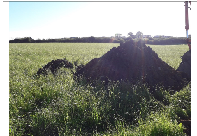
Trial Pit 101 Spoil
