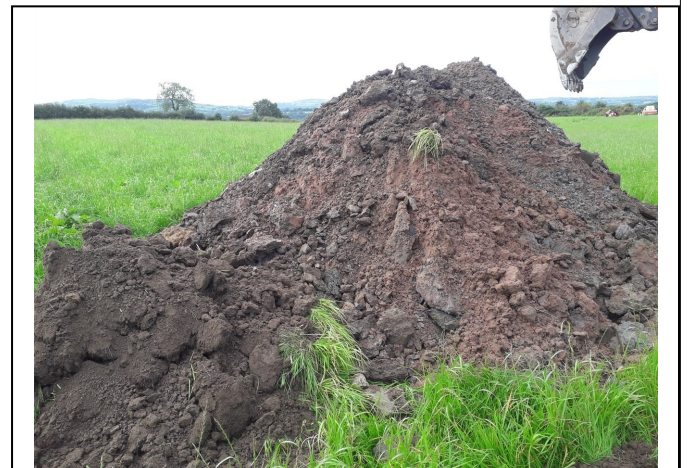
Trial Pit 120 Spoil
