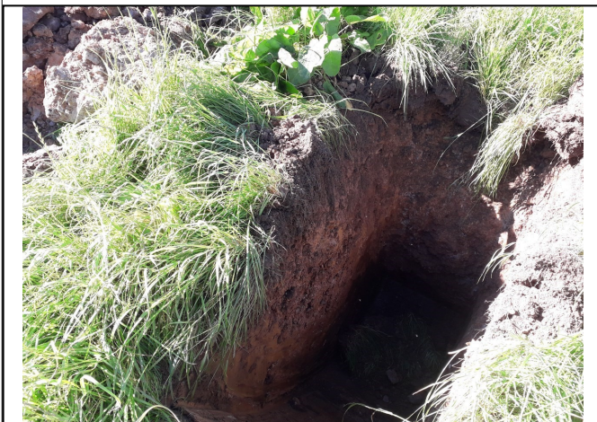
Trial Pit 108/ Soakaway 104
