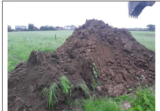
Trial Pit 130 Spoil
