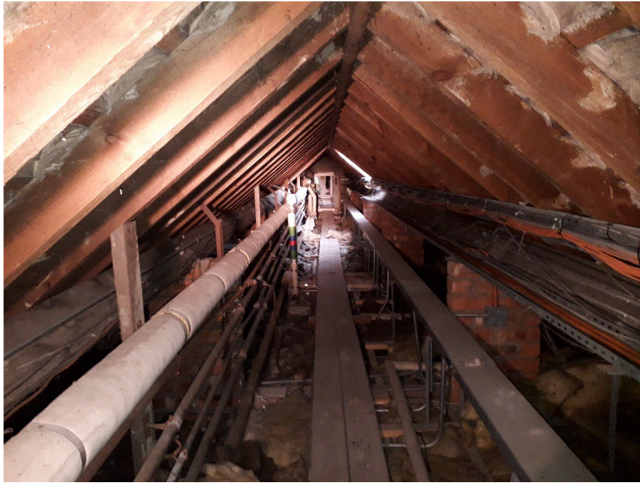
Plate 19. Roof void 2 access from void 3.
