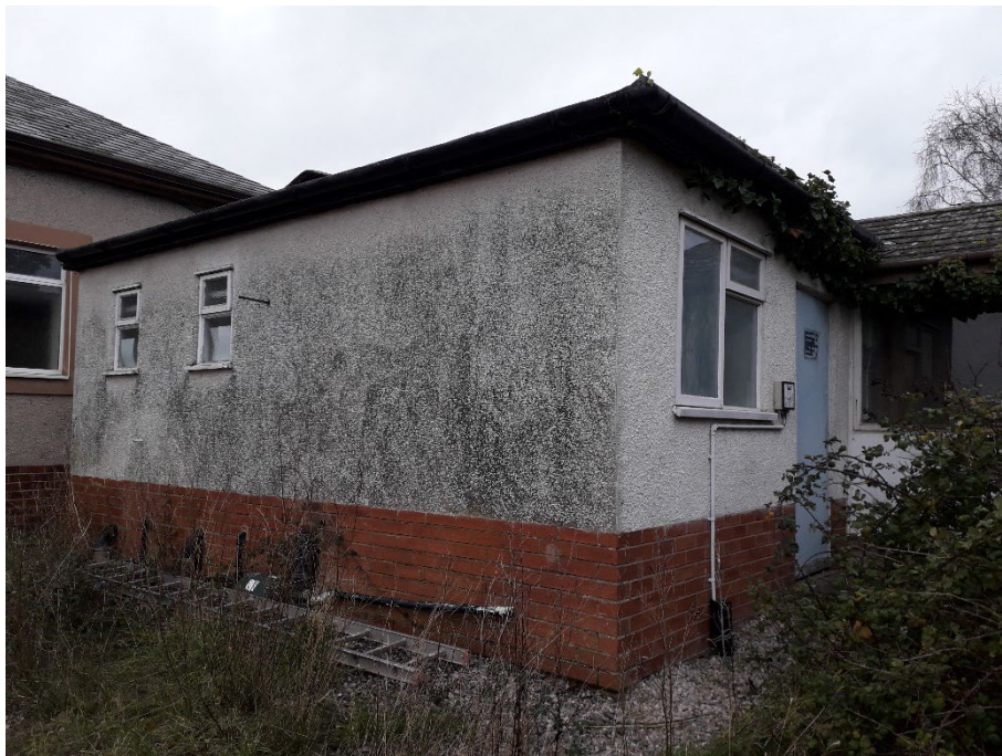
Plate 26. Building joining Building E to Buildings B and C.
