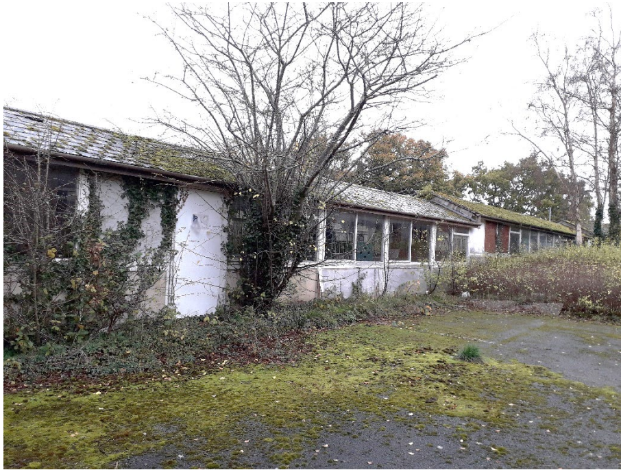
Plate 25. Western elevation of the building.
