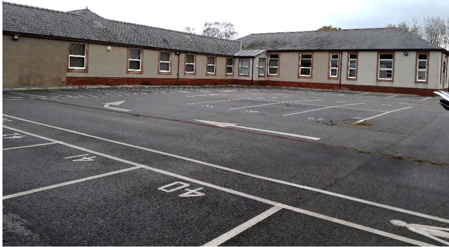
Plate 15. South-east elevation (rear) of the building.
