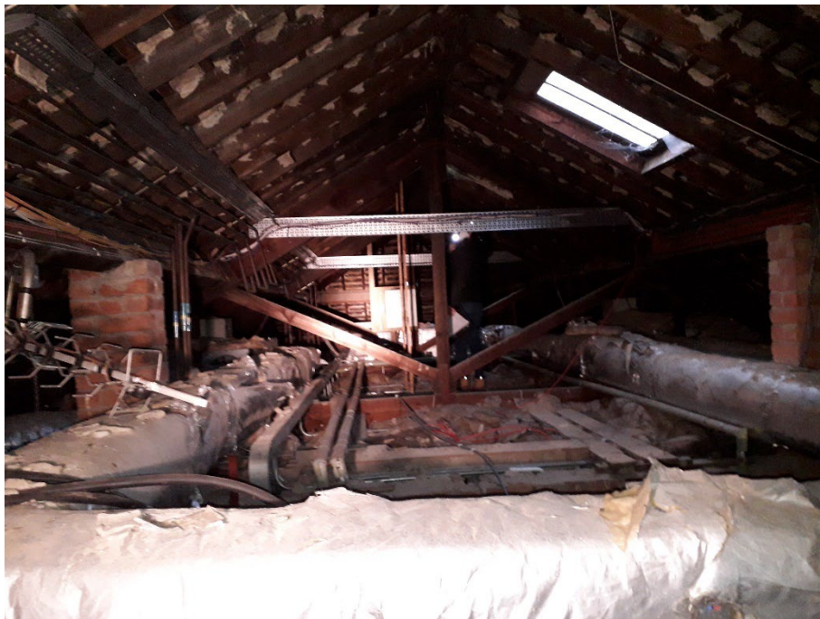
Plate 6. Internal view of roof void 1.
