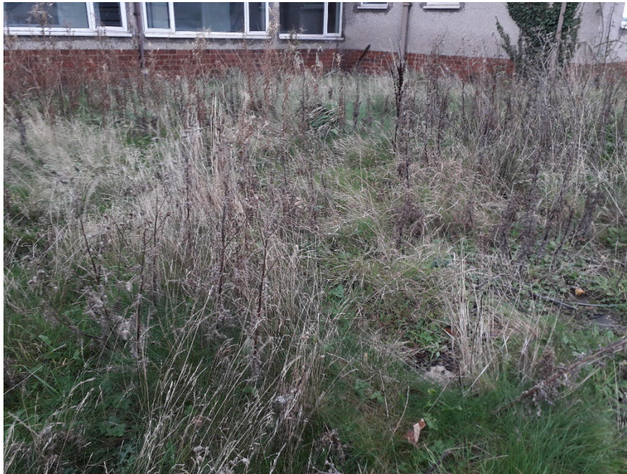
Plate 29. Unmanaged grassland at the front of Building A.
