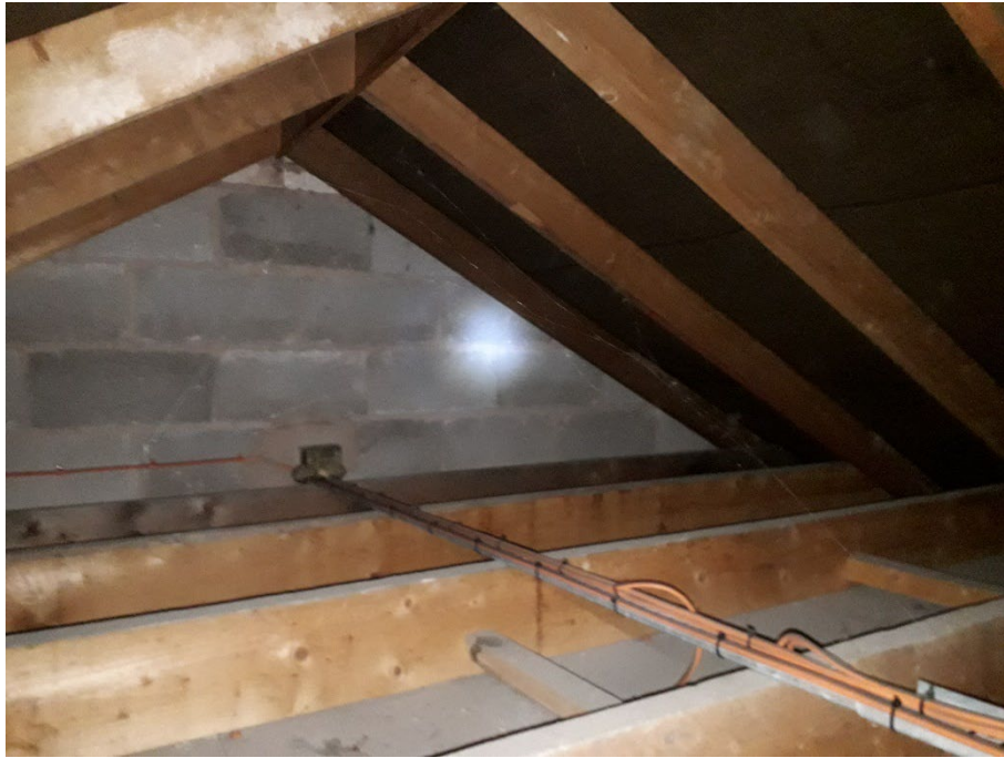
Plate 23. Example of roof void within the building.
