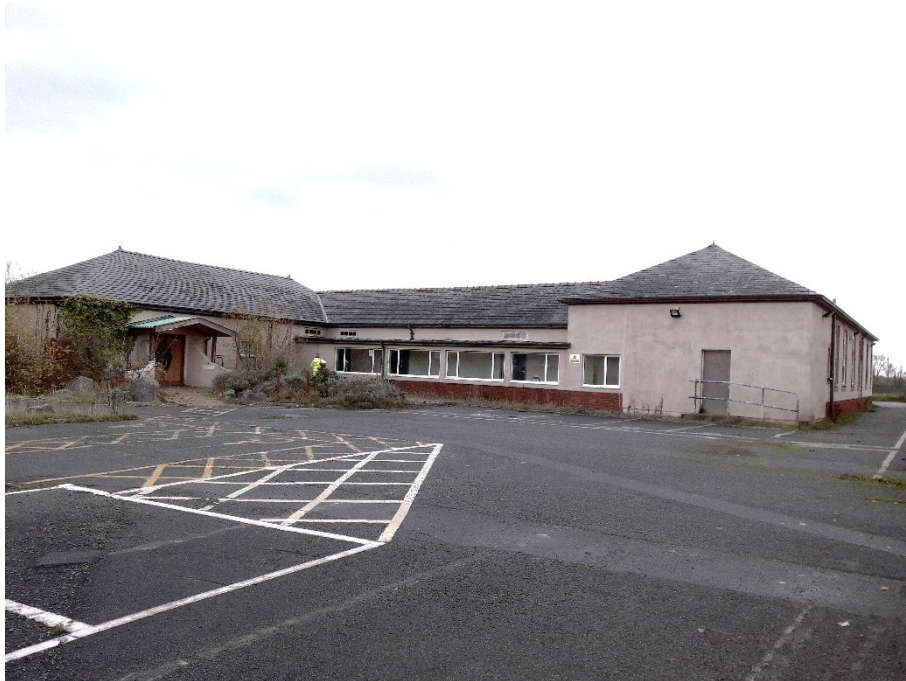
Plate 14. North-west elevation (front) of the building.
