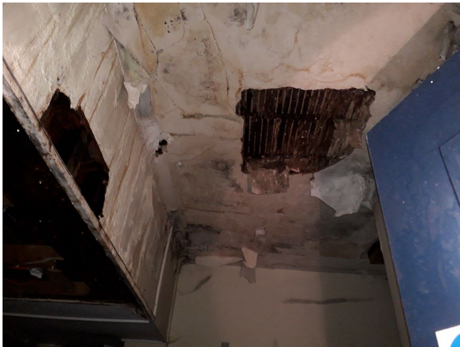
Plate 18. Ceiling below roof void 1 and part of 2.
