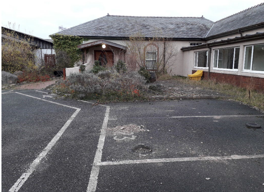
Plate 34. Amenity planting (introduced shrub) by the entrance of Building C.
