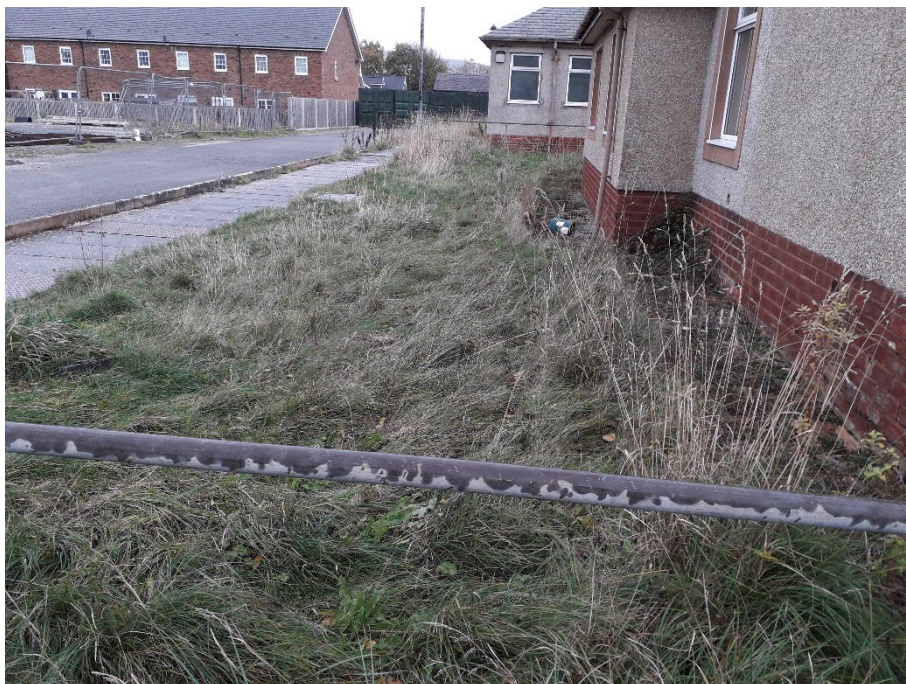
Plate 30. Unmanaged grassland at the front of Building A.
