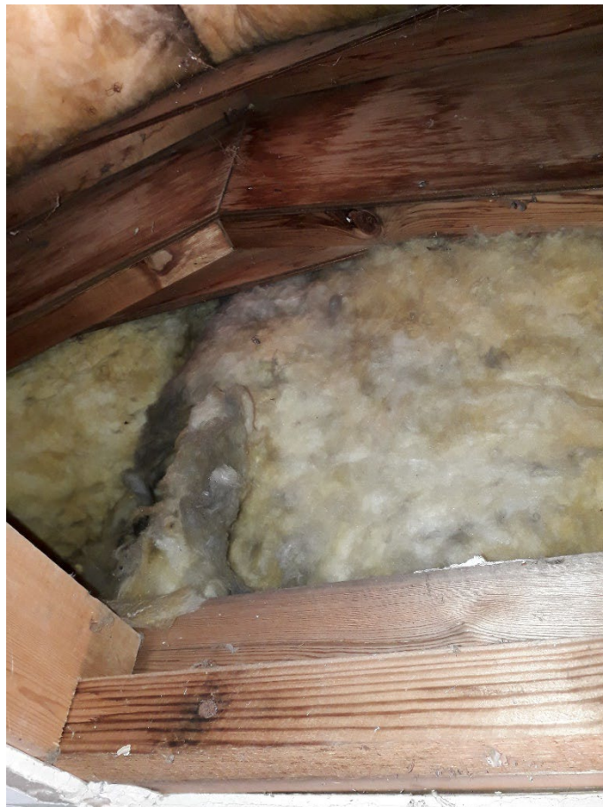
Plate 28. Example of roof void filled with insulation.
