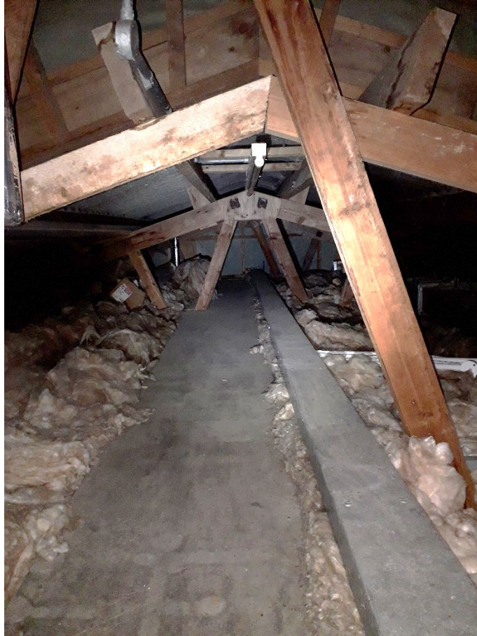
Plate 13. Internal view of small roof void.
