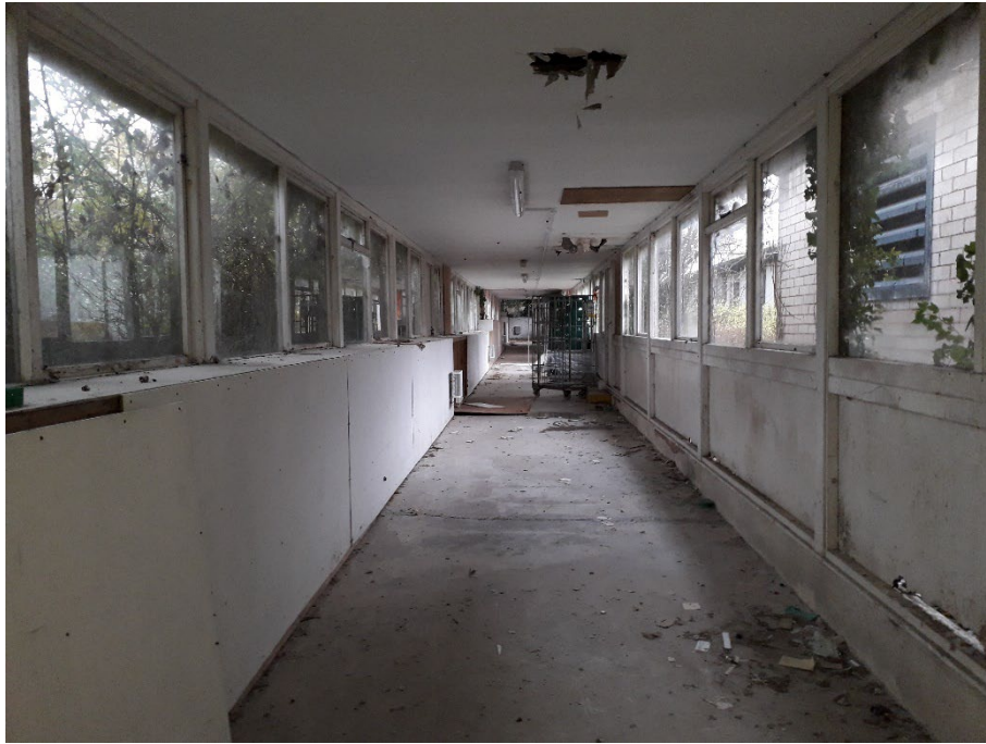
Plate 27. Internal view of Building E.
