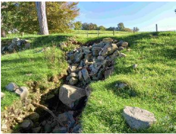
Photograph 15: Stone pile (TN3)
