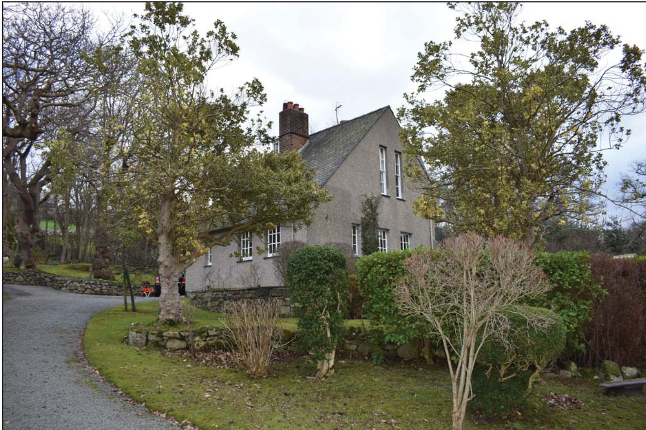
Plate 05: North-northeast and west-northwest facing elevations of Wern Isaf (LB3567) (viewed from the northwest; archive ref G2757_SA_011).
