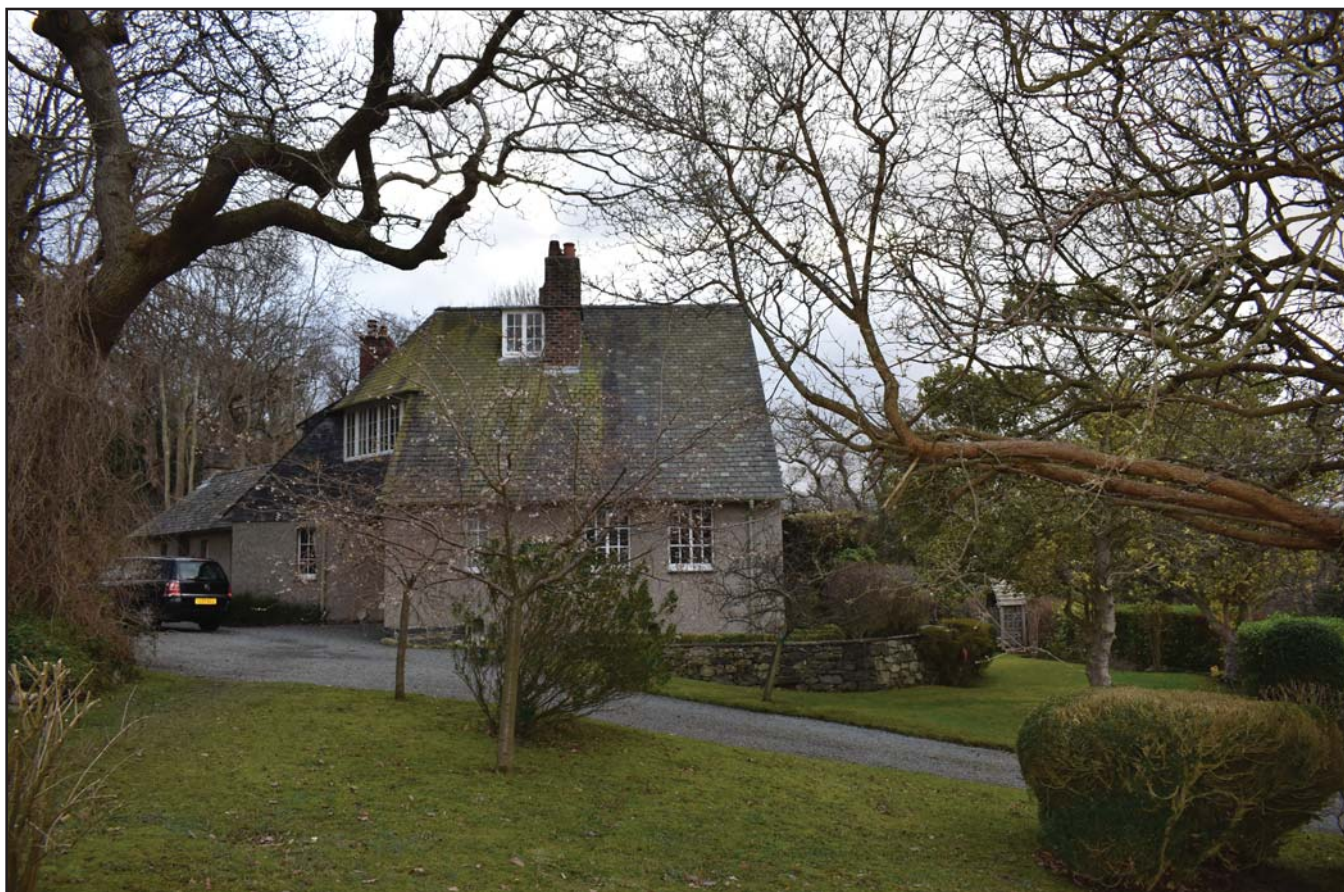
Plate 06: North-northeast facing elevation of Wern Isaf (LB3567) (viewed from the north-northeast; archive ref G2757_SA_012).
