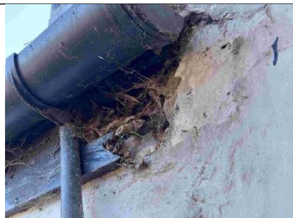
Photograph 4: Eastern elevation of B1. Large gaps present between facias and walls
