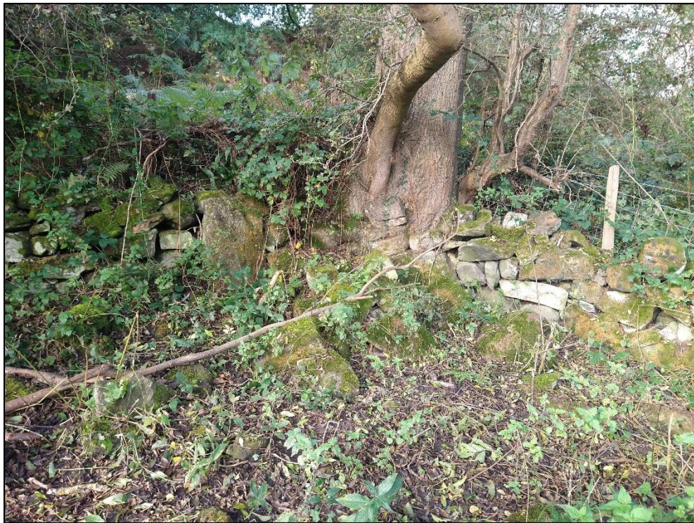
Plate 6: TN5 – Dry stone wall on the western site boundary.
