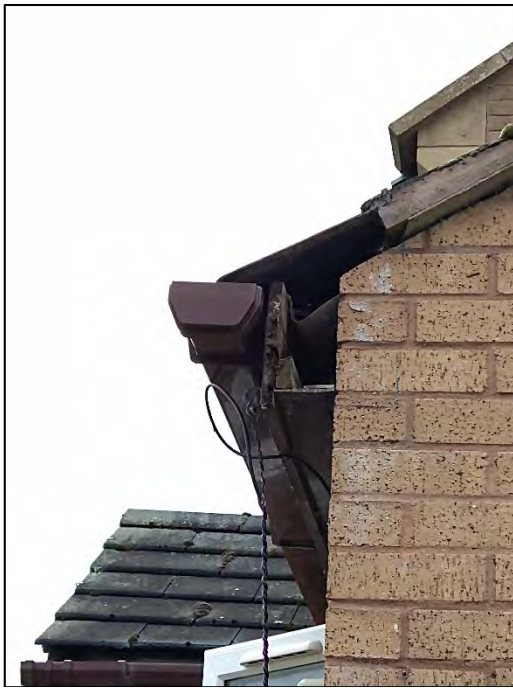
Plates 11 & 12: Examples of Potential Roost Features for bats within structure of Building 3, consisting of open soffit boxes and lifted lead flashing.
