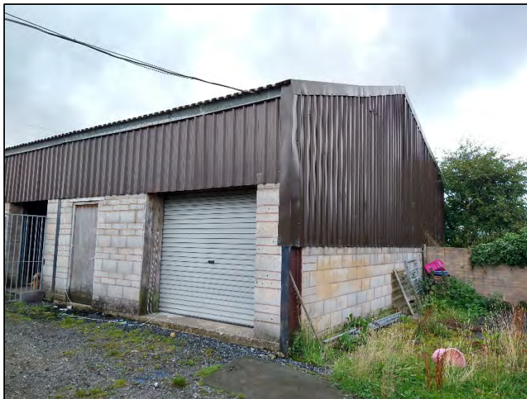
Plate 8: Exterior of Building 2.
