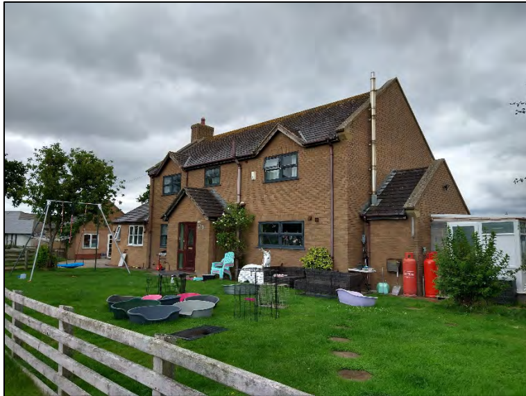
Plate 10: Exterior of Building 3 (farmhouse) showing brick built construction, tiled roof and surrounding amenity grassland lawn.
