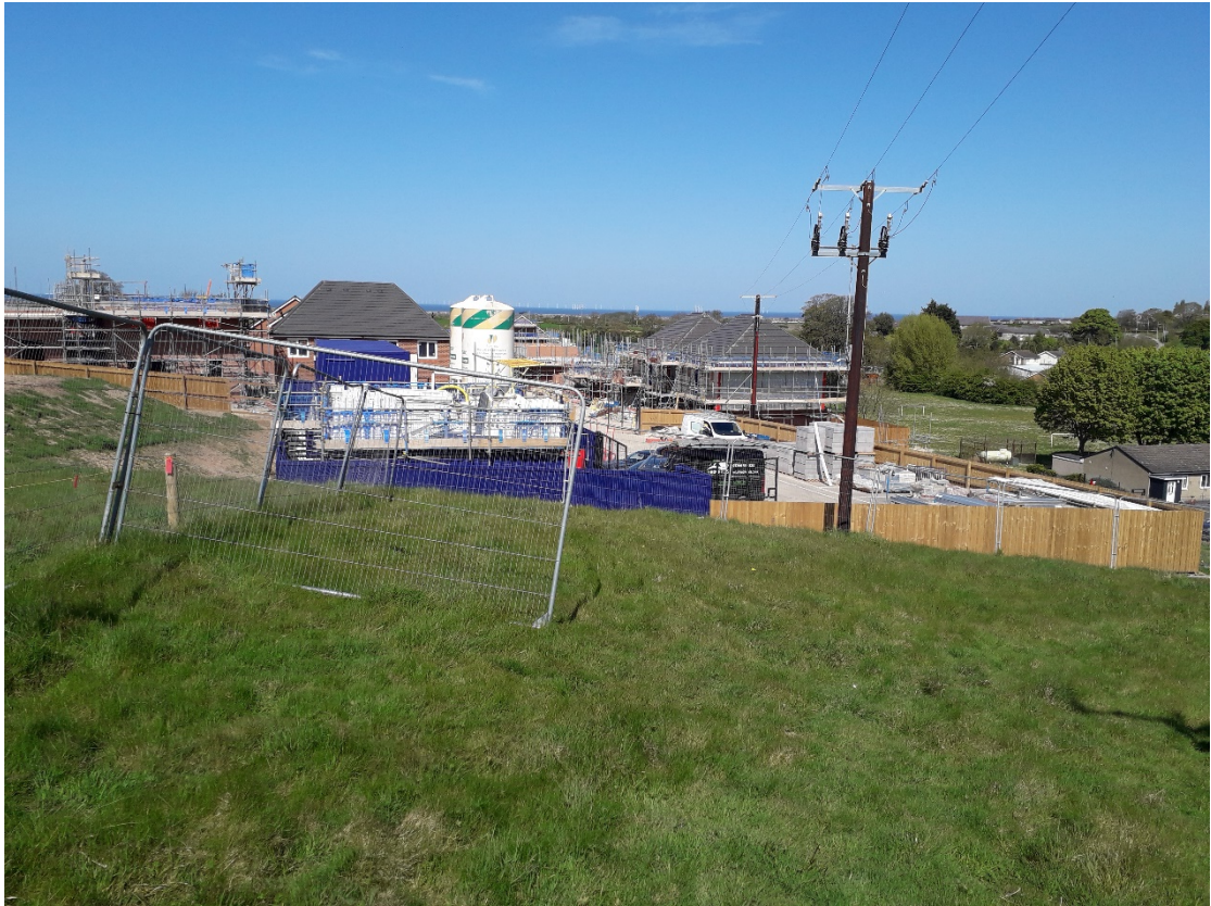
Plate 3. Looking north-west at Phase 1 and site compound.
